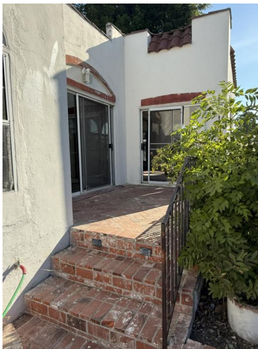
Photograph 5. Overview of south elevation sliding glass doors, view east.
