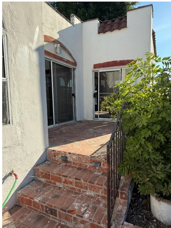
Exhibit 7. Overview of south elevation sliding glass doors, view east.
