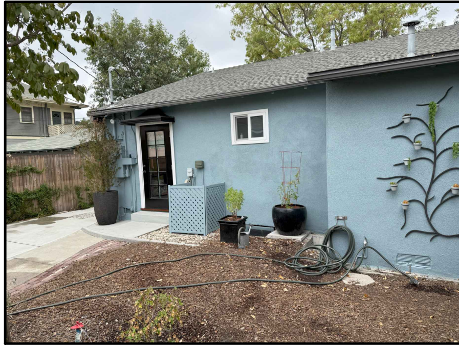
EAST ELEVATION - AREA OF HOUSE WHERE ADDITION WILL BE ADDED.
