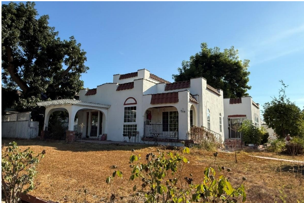
Exhibit 3. West elevation, view northeast.
