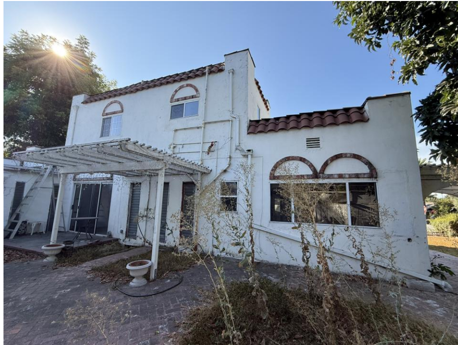
Photograph 8. Overview of north (rear) elevation exterior with two-story section, view south.
