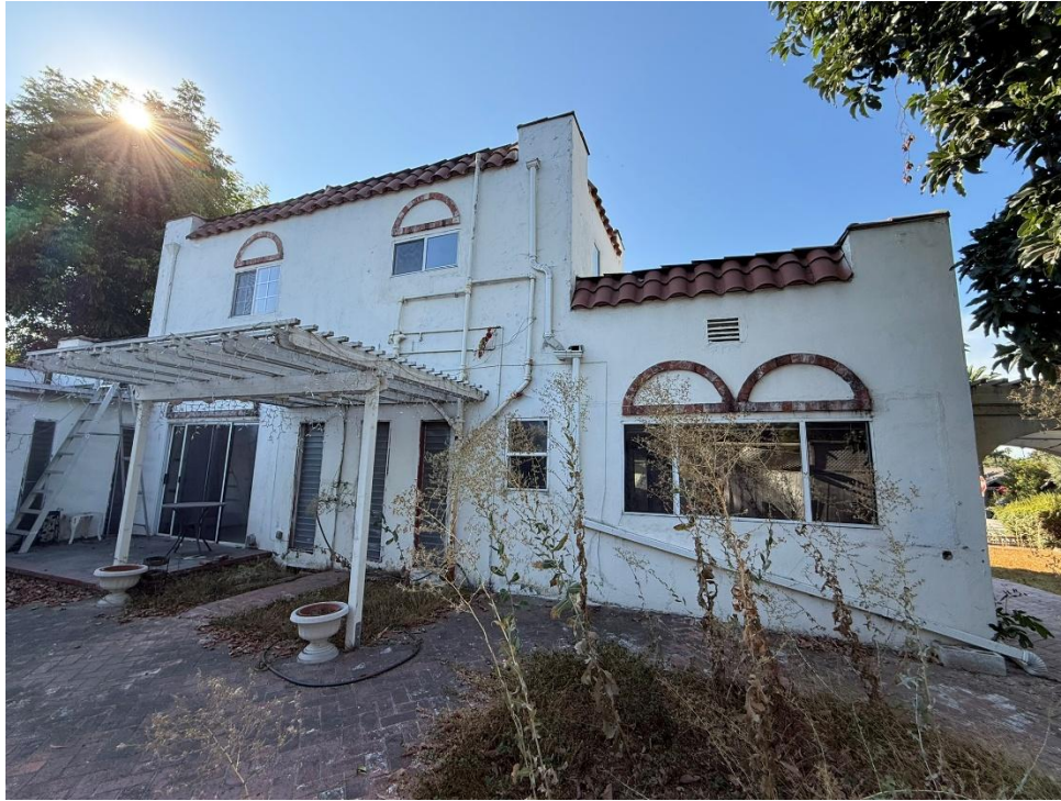
Exhibit 10. Overview of north (rear) elevation exterior with two-story section, view south.
