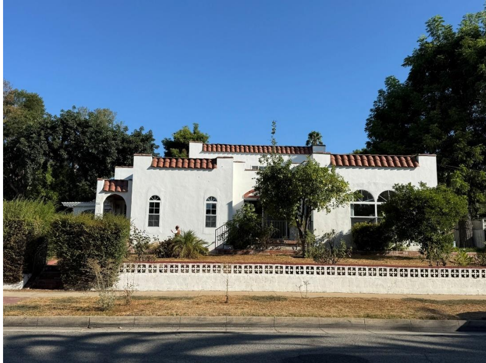
Exhibit 6. Overview of south elevation, view north.
