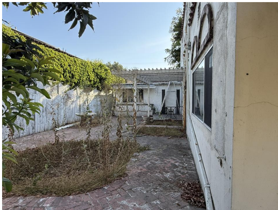
Photograph 7. Overview of north (rear) elevation, view east.
