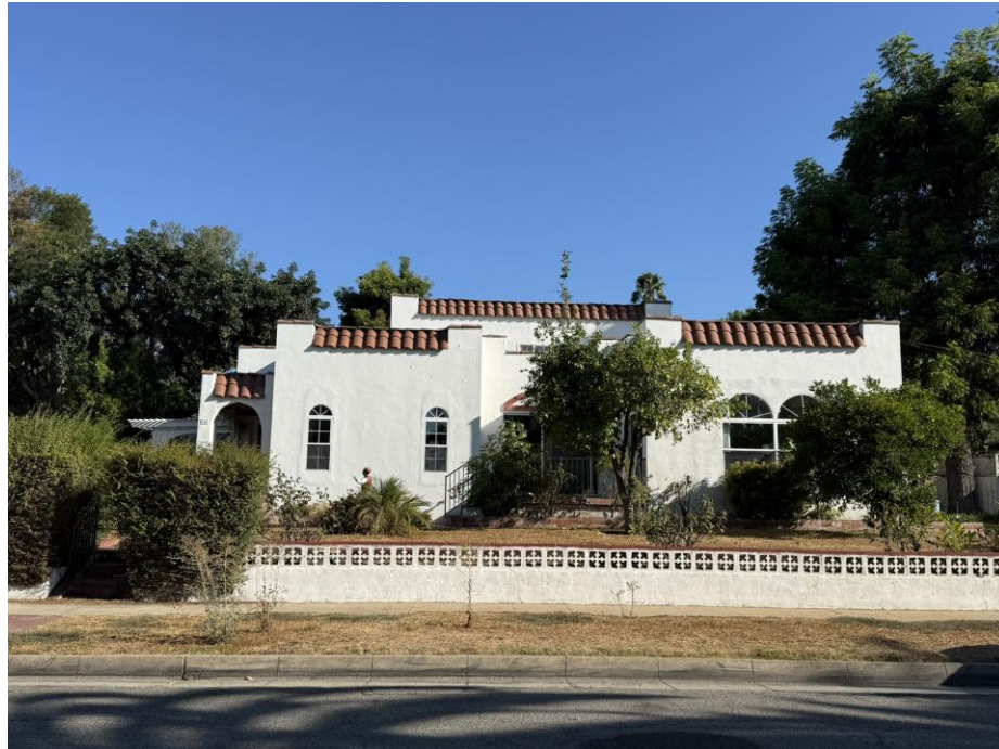
Photograph 4. Overview of south elevation, view north.
