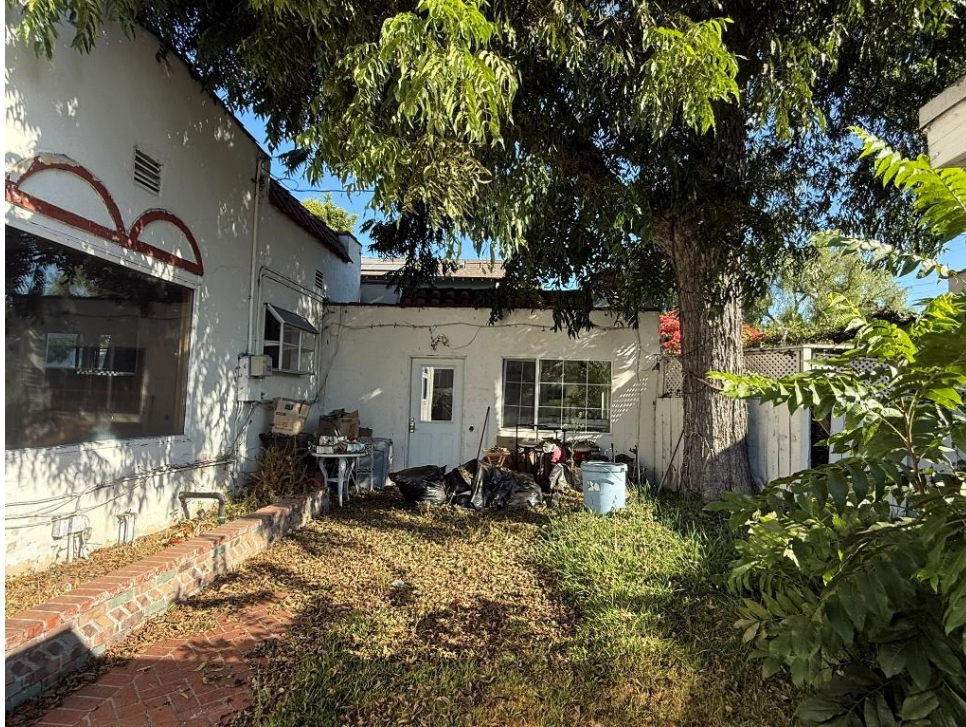
Exhibit 8. Overview of east elevation, view north to the garage-turned-addition.
