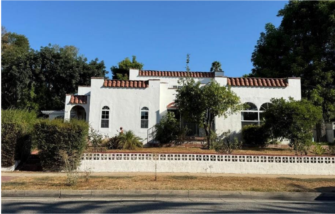
Image 3: 644 Stratford Avenue – South Elevation
