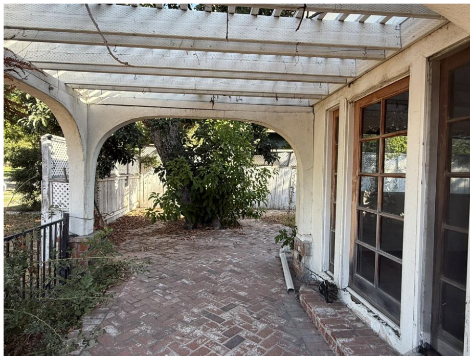
Photograph 3. Overview of west elevation pergola, view north.
