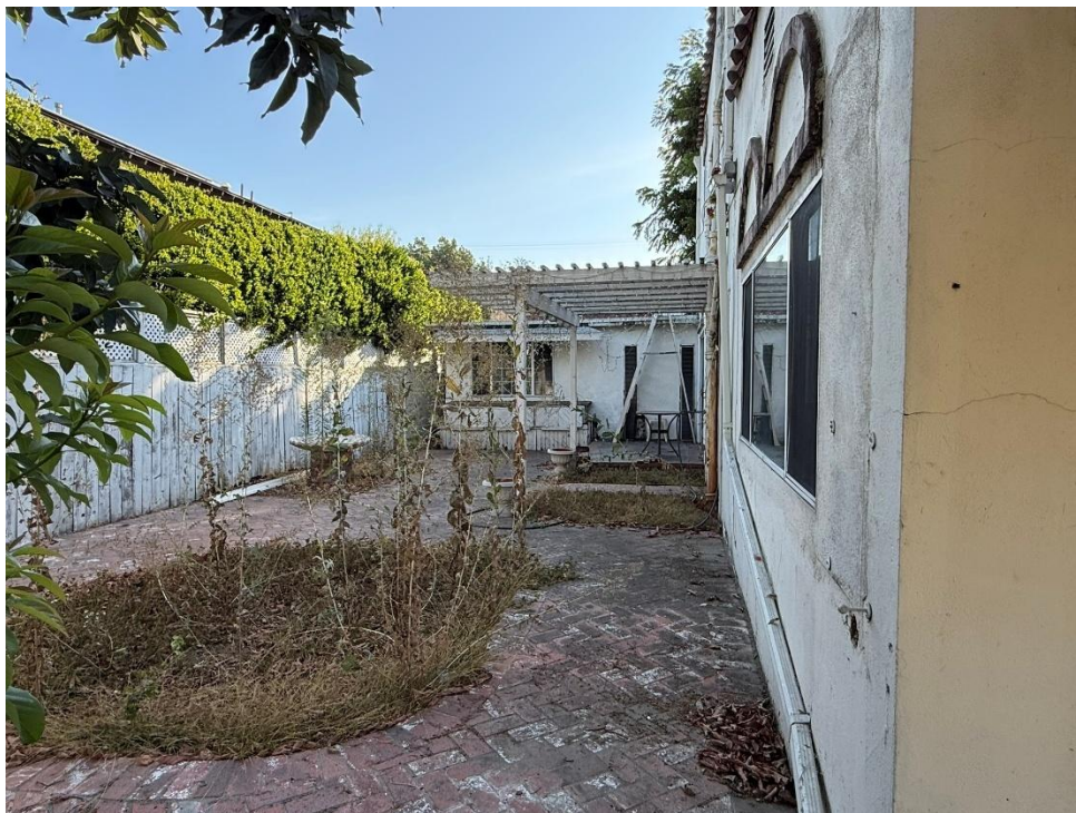
Exhibit 9. Overview of north (rear) elevation, view east.
