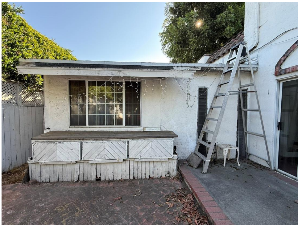
Exhibit 11. Overview of garage-turned-addition, view east.
