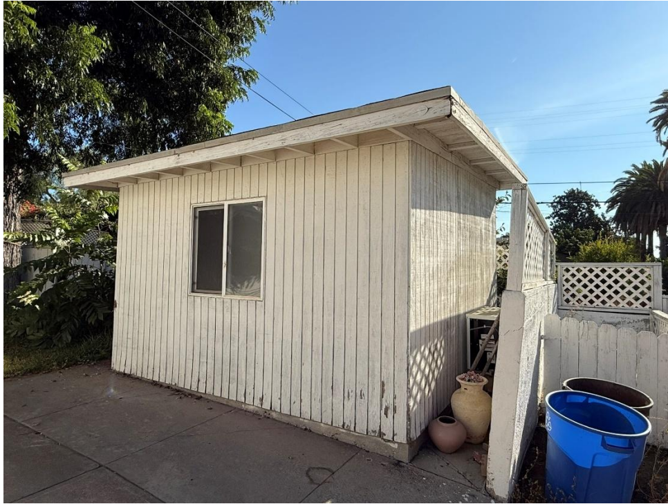
Exhibit 12. Overview of ancillary building, view east.
