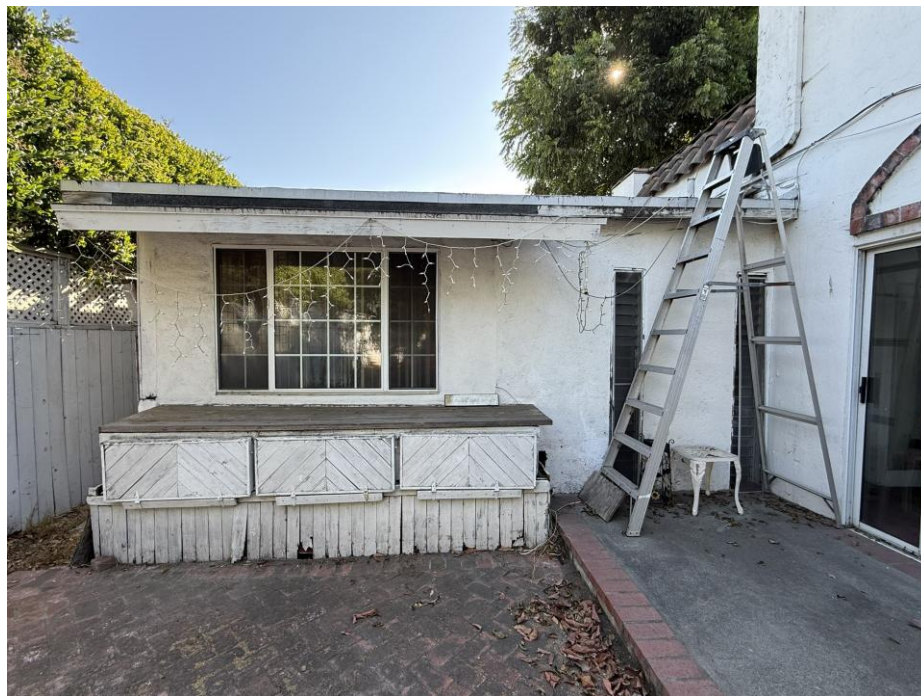
Photograph 9. Overview of garage-turned-addition, view east.
