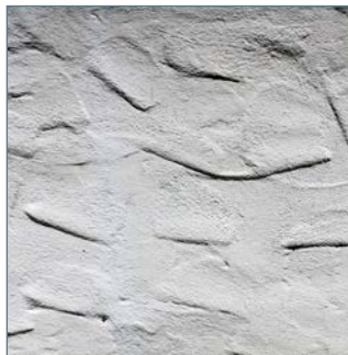
Stucco with different trowel patterns
