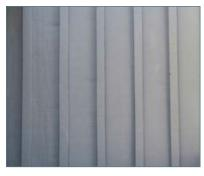
Vertical wood board-and-batten siding
