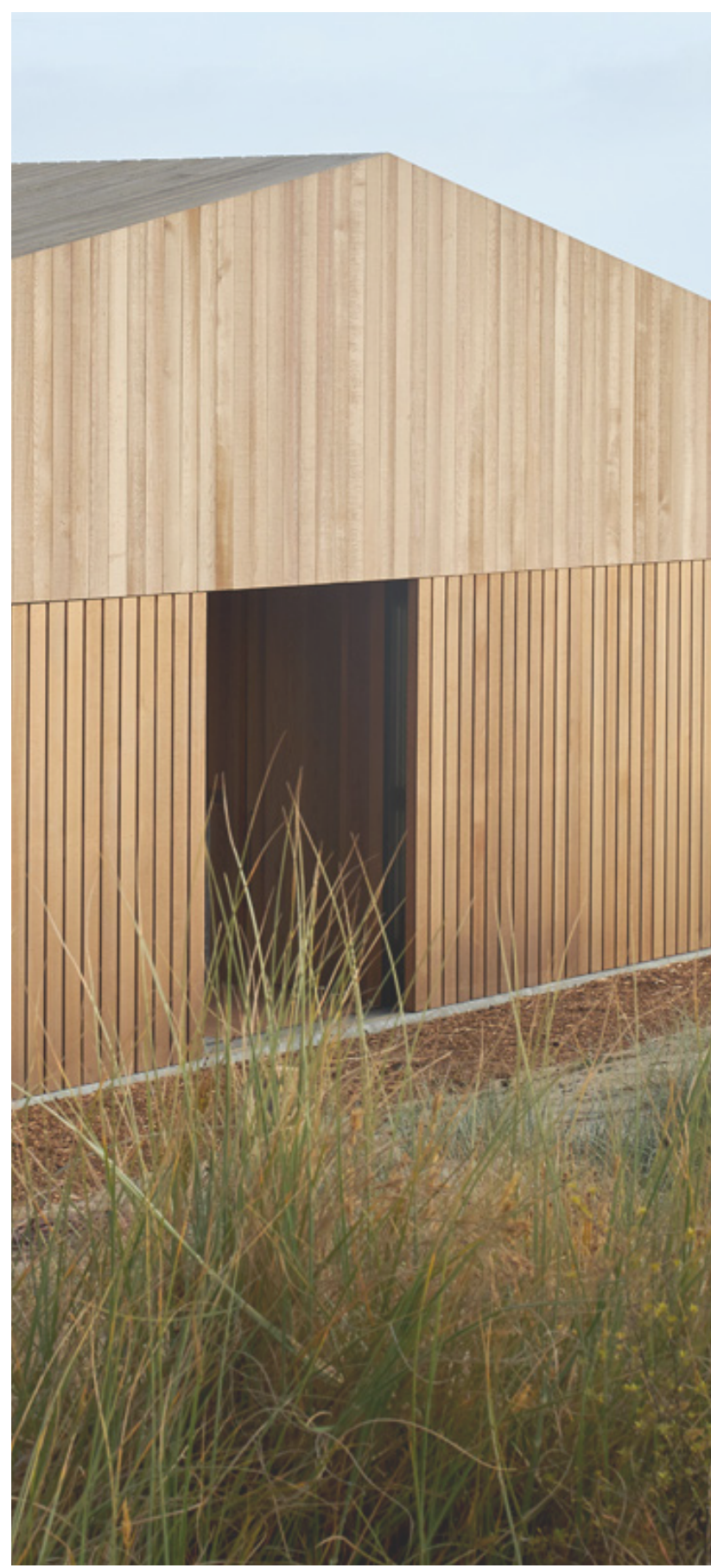
WOOD SIDING 4"-5" VERTICAL BOARD, SET WITH 1/8" GAP. SMOOTH FINISH. LIGHT BROWN STAIN WITH NATURAL VARIATION AND MATTE FINISH COAT
