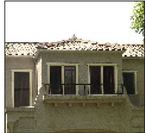
Roofs are a visual element of the building: materials and roof pitch contribute to character.
