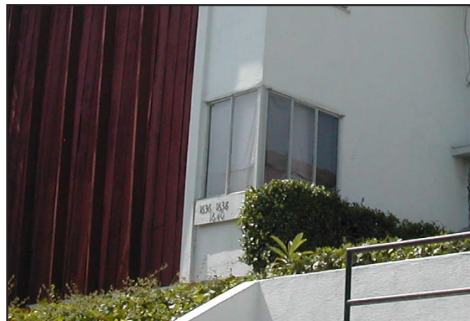
A corner window of a multi-family unit.
