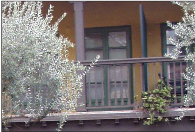
Balconies are common features and often the doors to these areas are character-defining features.
