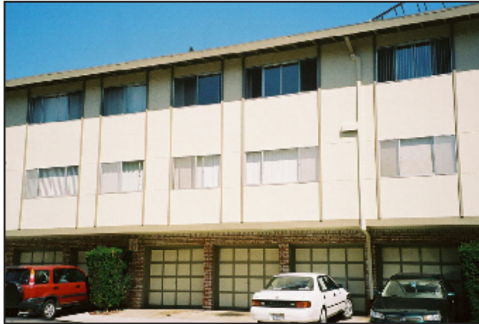
We can learn lessons from past failures in multi-family design.
