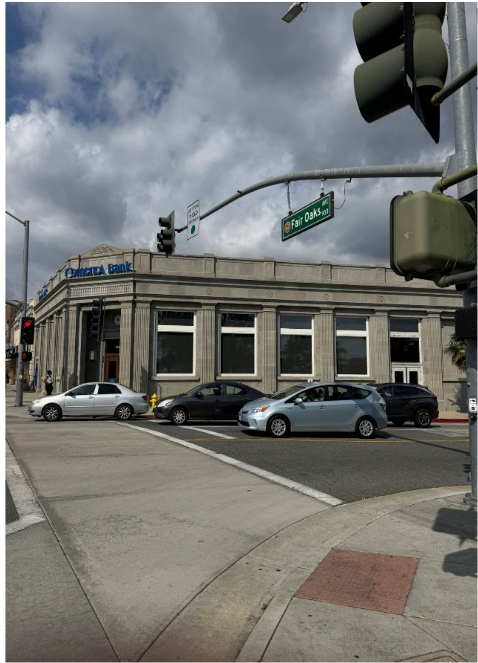
Photo 41 Radius Map Reference: 41 Site Address: 820 Fair Oaks Ave Site City: South Pasadena Site ZIP: 91030 APN: 5318-014-001 Property is located within 300-foot radius of site subject.
