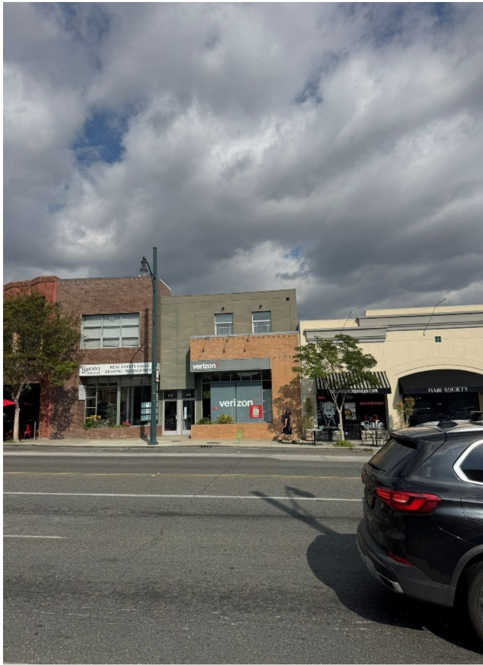
Photo 42 Radius Map Reference: 42 Site Address: 818 Fair Oaks Ave Site City: South Pasadena Site ZIP: 91030 APN: 5318-014-003 Property is located within 300-foot radius of site subject.
