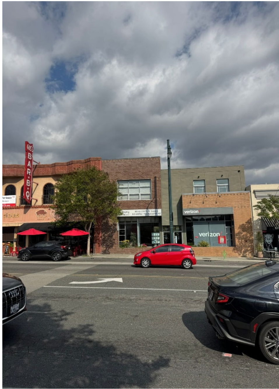
Photo 43 Radius Map Reference: 43 Site Address: 814 Fair Oaks Ave Site City: South Pasadena Site ZIP: 91030 APN: 5318-014-096 Property is located within 300-foot radius of site subject.
