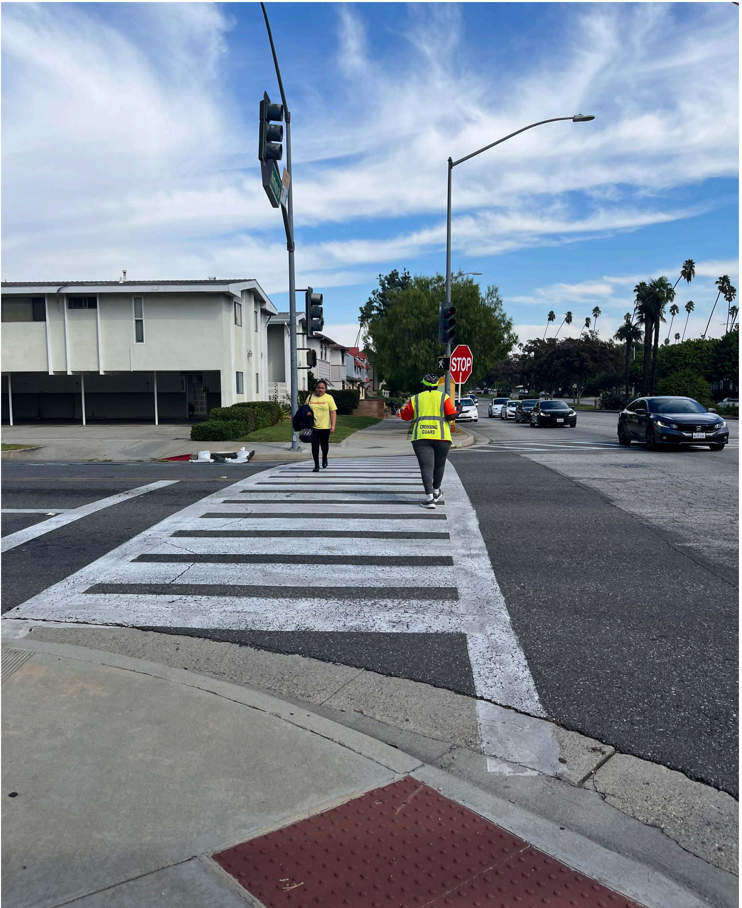
Figure 3: Existing Pedestrian Crossing at Huntington Drive
