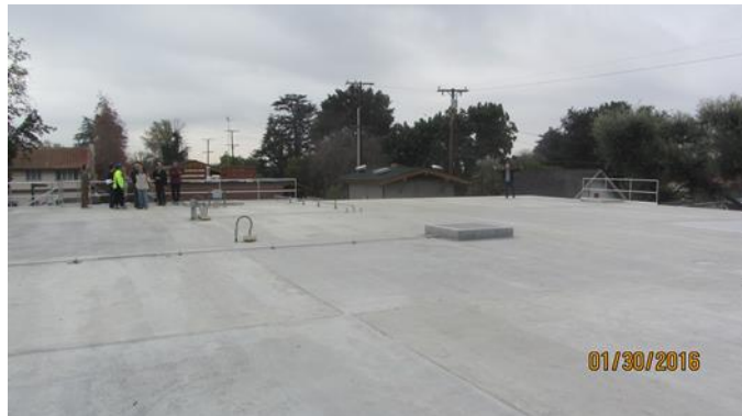
Figure 4: Site Visit to Wilson Reservoir. Note the new concrete roof structure.
