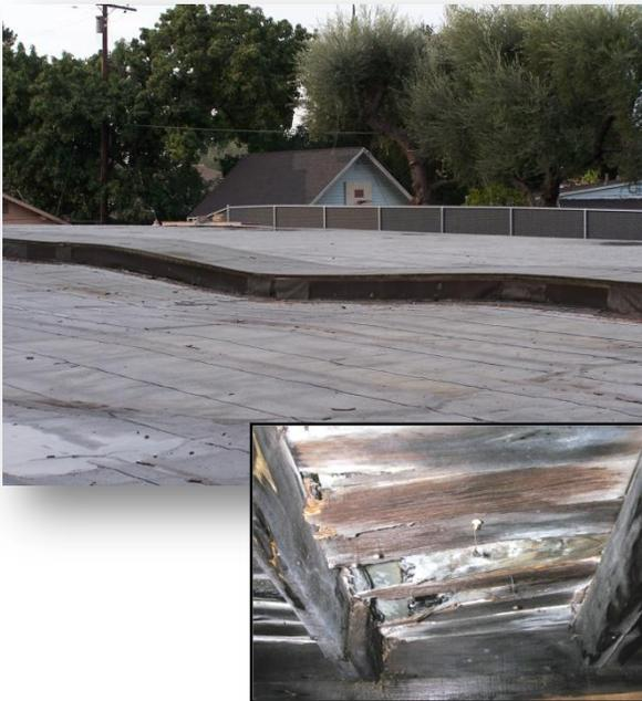
In recent years, the roof of the 90-year-old reservoir has begun to deteriorate and sag in areas. An inspection in early 2008 concluded that a severe roof collapse could occur at any time. Because of its age, the reservoir also does not meet current earthquake resistance standards. For these reasons, the inspection report recommended complete replacement of the reservoir.
